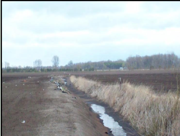
Lake Smith Drain No. 2— northeast of Greenway Drive. No vegetated buffer strip and topsoil entering and filling the drain.
