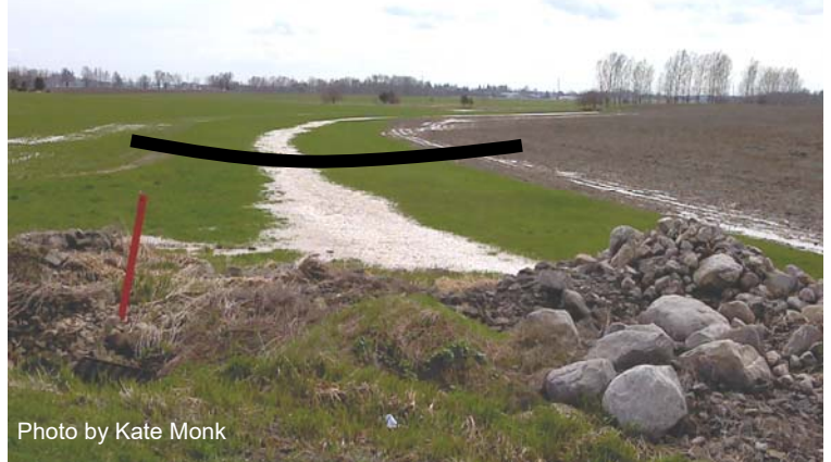
The saucer shape of the grassed waterway guides water to where you want it to go
